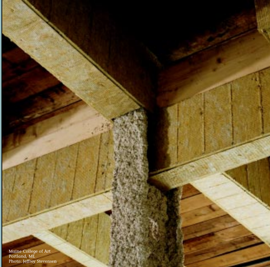
Conventional cementitious fireproofing on column. Beams protected with Albi DriClad.
