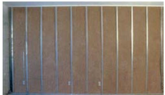
Celbar completely and uniformly fills wall cavities
