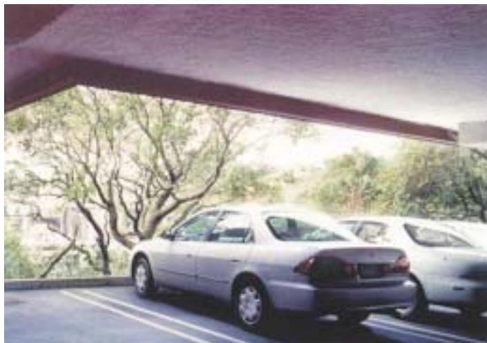
*K-13 sprayed to this concrete parking deck provides thermal control to the conditioned spaces above.*
